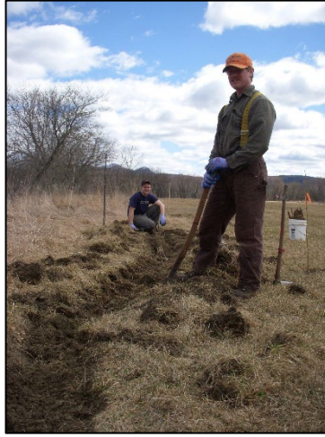
FIGURE 2: FASCINE TRENCH MAKING
