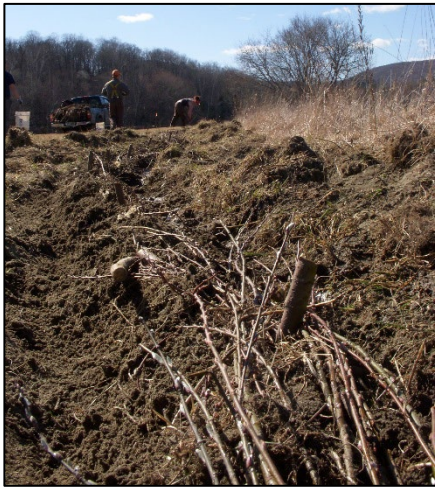
FIGURE 3 & 4: FASCINE INSTALLATION
