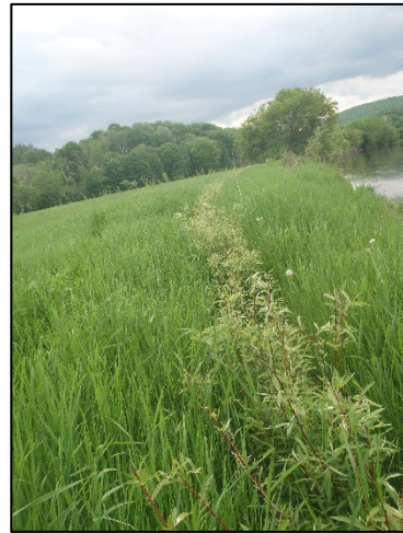
FIGURE 5: FASCINE AFTER ONE YEAR OF INSTALLATION
