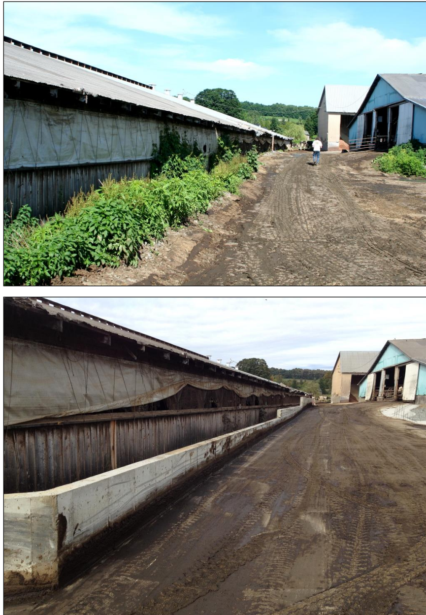
Figure 34. The Gray Farm undertook numerous clean water diversion and runoff control projects in 2015 and 2016 to improve water quality conditions in a tributary of Stearns Brook. The top photo shows a barnyard area prior to construction on 3 July 2015, and the bottom photo shows the same area during construction of a barrier to separate clean and contaminated water on 28 September 2015 (bottom photograph courtesy of Ben Copans).
