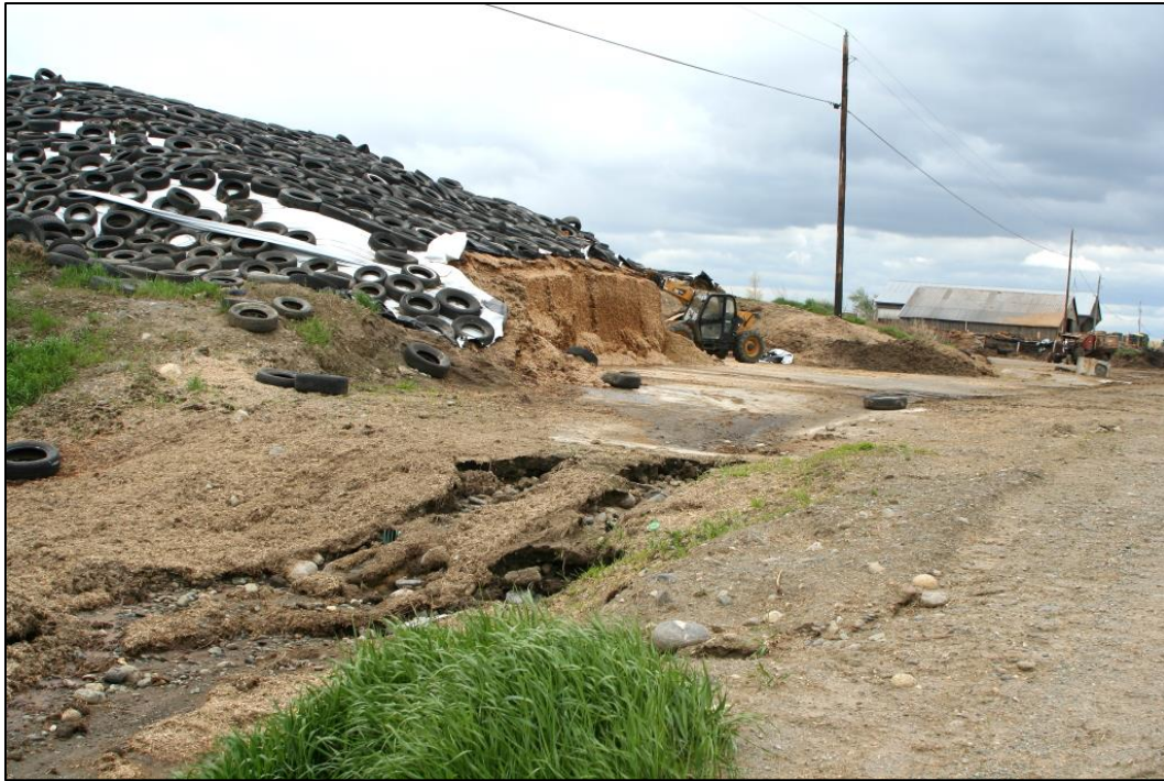
Figure 54. When debris plugs the drain, leachate from this silage storage pad flows into a roadside ditch and then into Alder Brook, a tributary of the Barton River. Note the soil erosion indicating the large quantities of water that flow into the roadside ditch and then Alder Brook.
