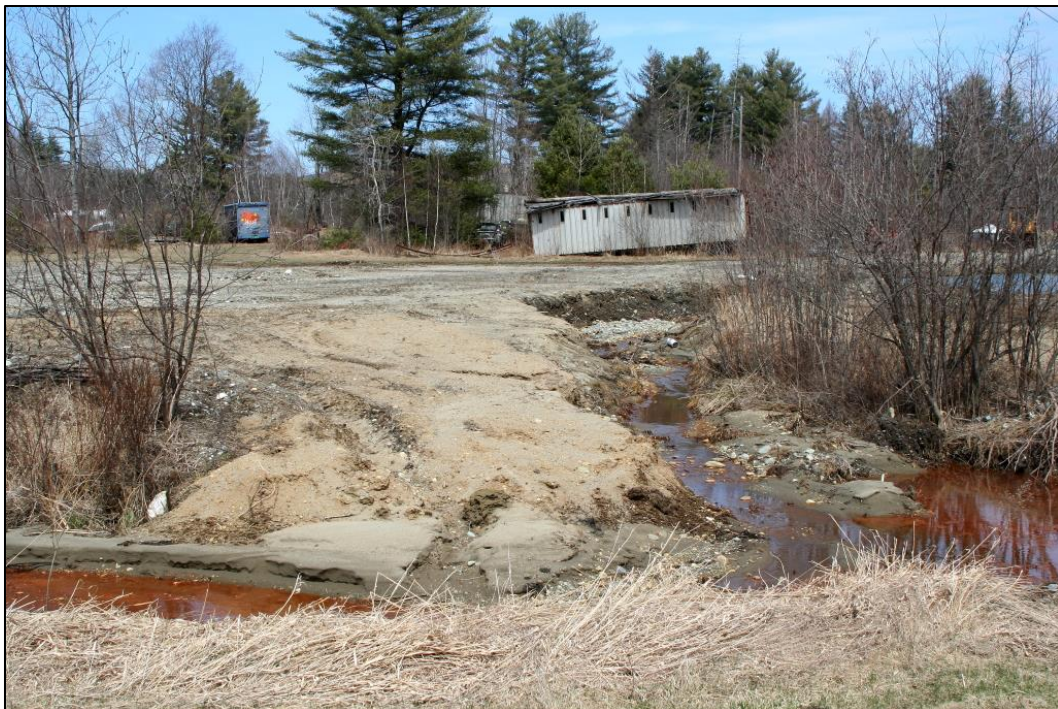
Figure 46. Area where wetlands had been excavated and filled along Nadeau Road in Coventry, Vermont.
