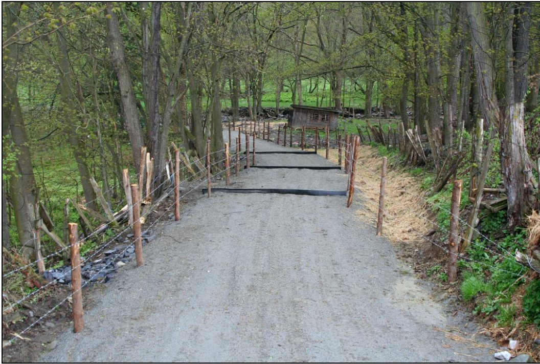
Figure 49. Hardened laneway and water barriers installed on a small dairy farm in Albany, Vermont to reduce runoff flowing into Shalney Branch (in background).
