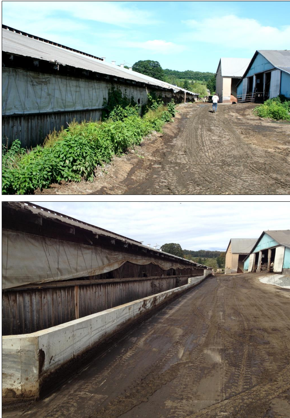
Figure 16. The large farm along the Tributary of Stearns Brook undertook numerous clean water diversion and runoff control projects during 2015-2017 to improve water quality conditions in the Tributary of Stearns Brook. The top photograph shows a barnyard area prior to construction on 3 July 2015, and the bottom photograph shows the same area during construction of a barrier to separate clean and contaminated water on 28 September 2015 (bottom photograph courtesy of Ben Copans).
