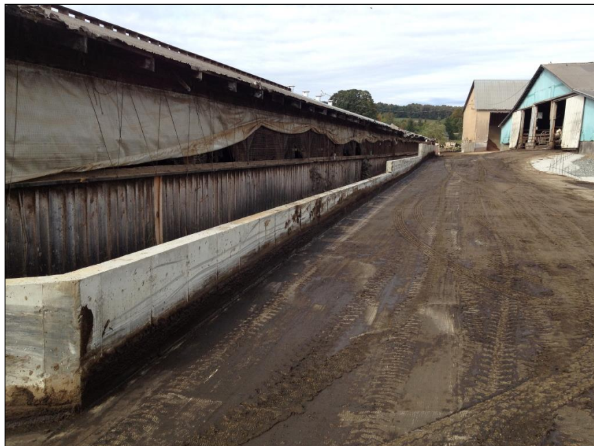
Figure 40. The Gray Farm undertook numerous clean water diversion and runoff control projects in 2015 to improve water quality conditions in a tributary of Stearns Brook. The top photo shows a barnyard area prior to construction on 3 July 2015, and the bottom photo shows the same barnyard area during construction of a barrier to separate clean and “dirty” water on 28 September 2015 (bottom photograph courtesy of Ben Copans).
