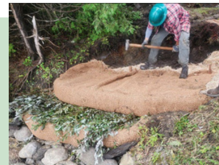
Encapsulated soil lifts installation Caspian Lake, 2023
